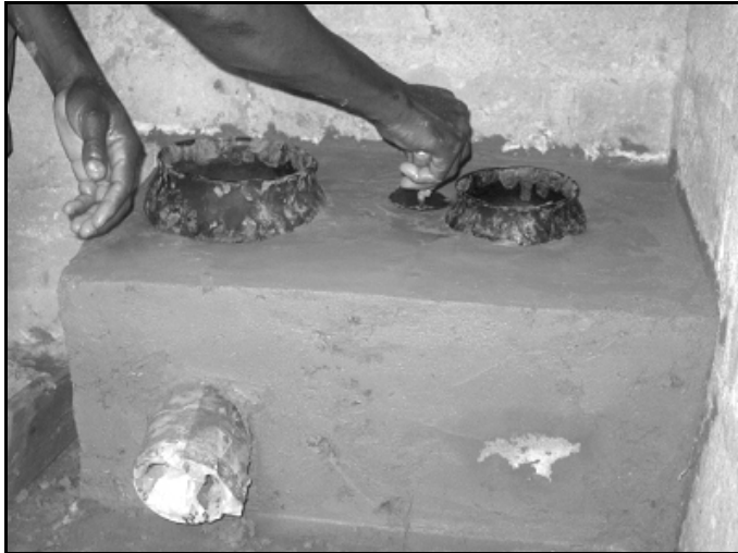
A village project co-ordinator building a rocket stove
